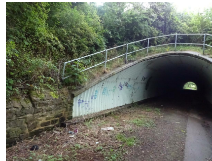
Photograph 2 (P2) West Entrance North end
