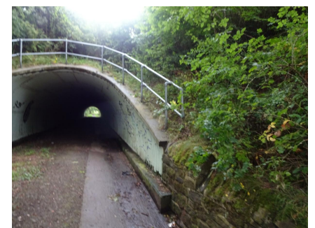
Photograph 3 (P3) West Entrance South end
