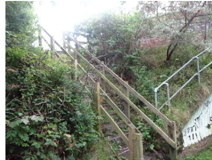
Photograph 6 (P6) East Entrance South end
